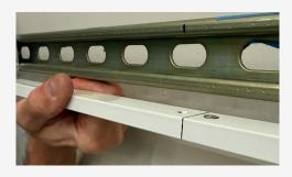
Push down on Axiom clip to engage completely to the grid. The fixture is now secured.
